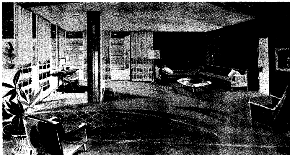
Stunning elegance Throughout the lobby begins in the lobby with carpeting by V'sosky, marble from Italy and Emerald Pearl Granite from Norway. The draperies
